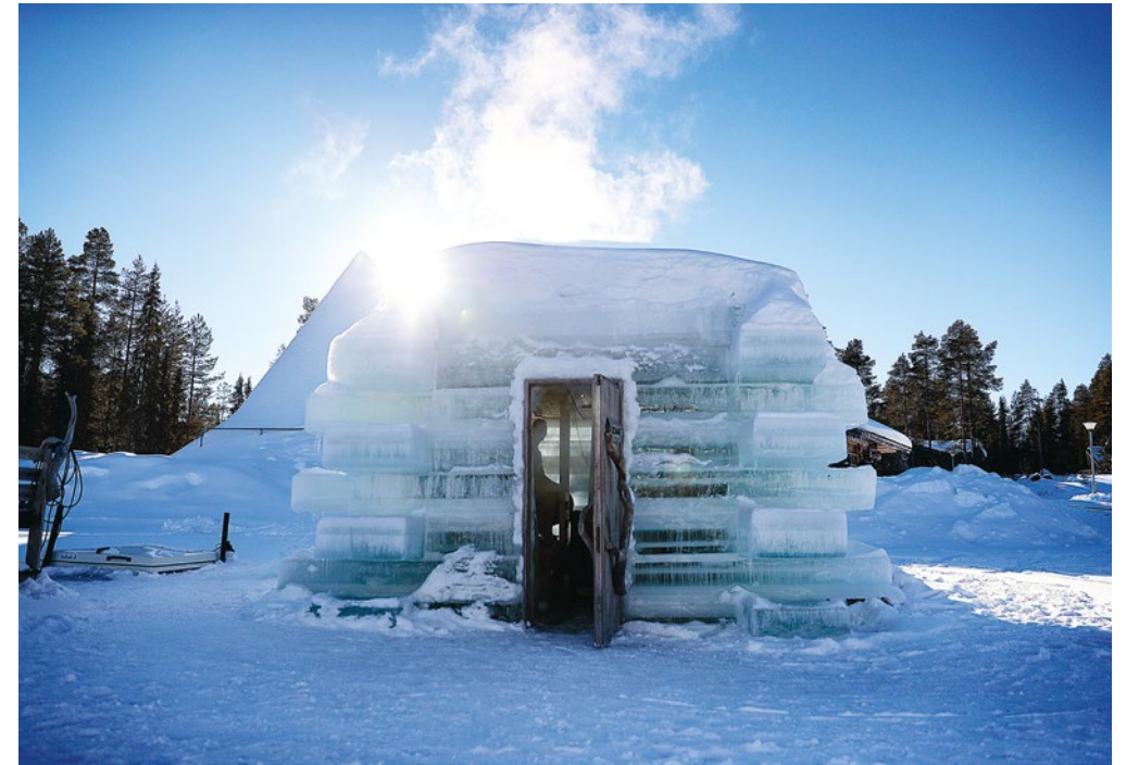
This winter sauna in Ruka, Finland, is constructed with ice blocks that create a humid sauna environment and simply melt back into the lake at the end of the season. Image © Visit Finland / Harri Tarvainen
