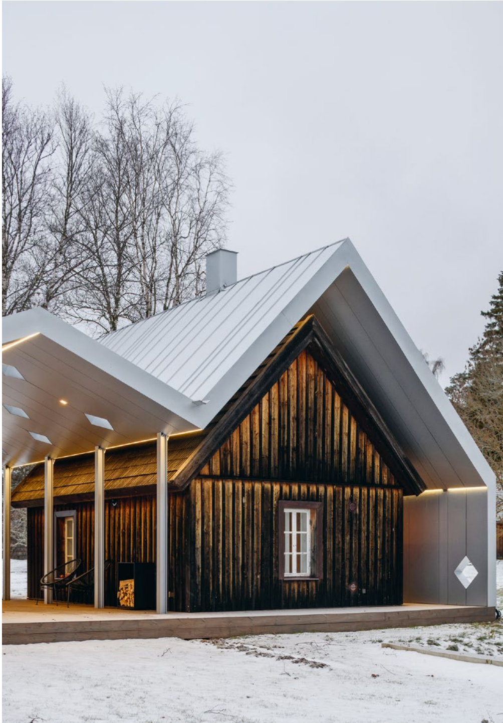
Lusthoone Sauna by Peeter Pere Arhitektid, Varbola Estonia, 2019. A new zig-zag roof protects the traditional sauna and creates sheltered exterior space. Image © Tõnu Runnel
