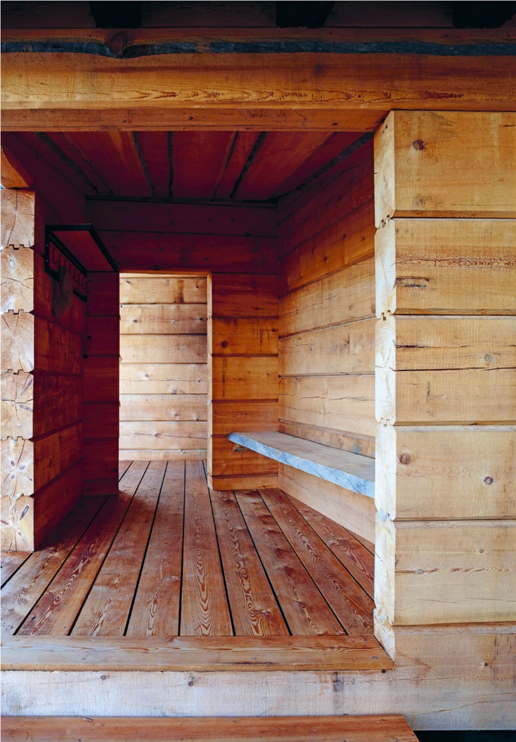
Massive wood with traditional jointing techniques at the Savusauna Joensuu by Tuomo Siitonen, Asikkala, Finland, 2016. Image © Rauno Traskelin
